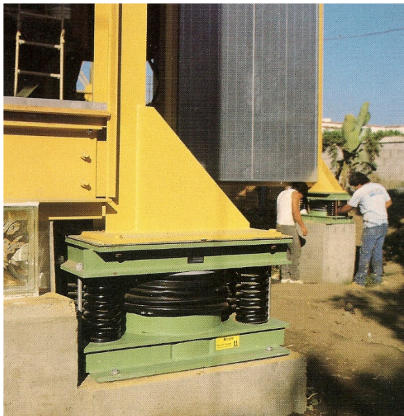
Figure 3. Three story building on springs in North Carolina to dampen earthquake waves. (Shustov, 1999)
