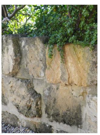
I used limestone blocks (approx. 40cm X 25cm X 10cm) to build retaining walls in my garden. I was restricted in size by what I could lift. Why did I not use granite for this retaining wall? Granite is much more dense/heavier. A block and tackle would be needed to lift granite blocks this size.
