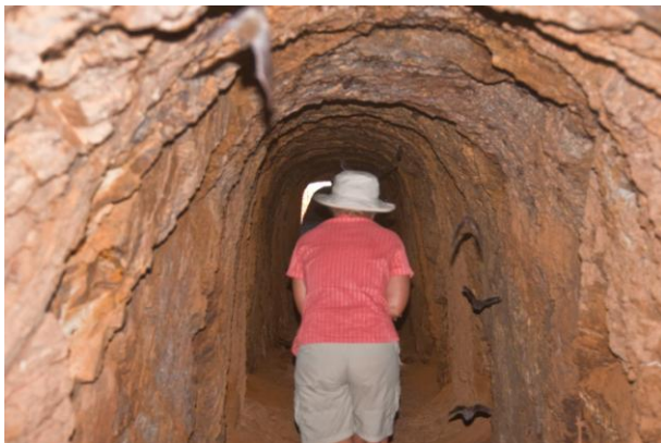
A gold prospector's adit driven into greenstones near Yalgoo. Note escaping resident micro-bats .
