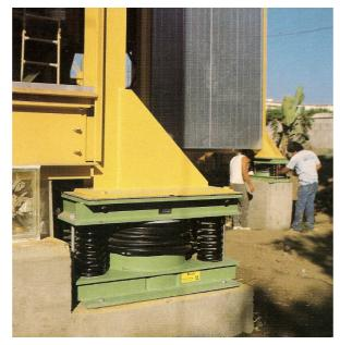
Figure 3. Three story building on springs in North Carolina to dampen earthquake waves. (Shustov, 1999)
